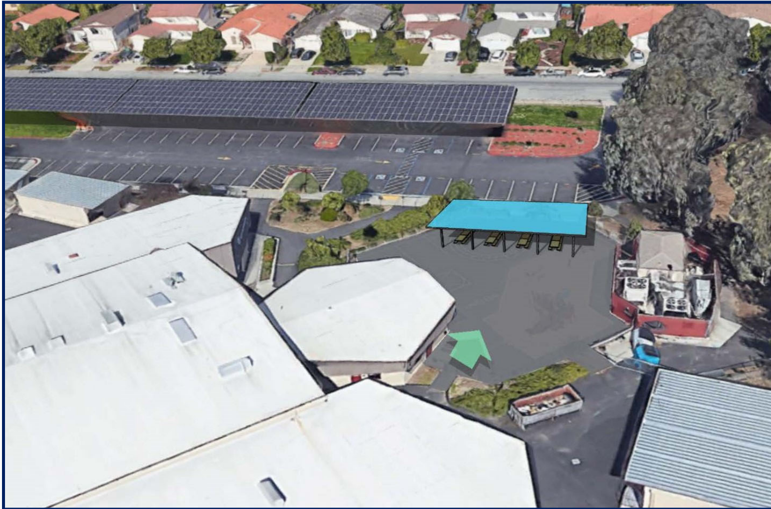
Cherrywood Shade Structure
